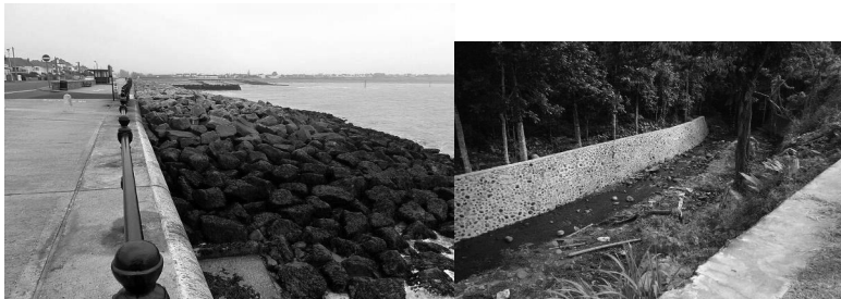
Rock armour revetments.
