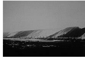
Overtopping on the inner slope of a dike in Northern during
